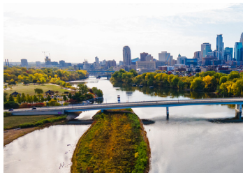
June 16, 2022 Hall's Island Restoration
