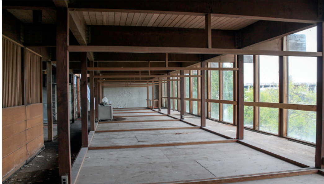
The upper floor prior to demolition, October 2017.
